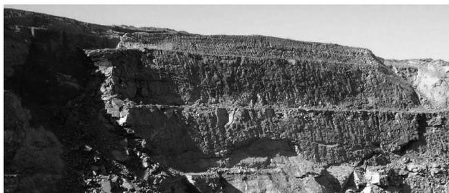
Figure 1 Photograph showing the RH28 pit slope failure on the northern wall of Round Hill pit
